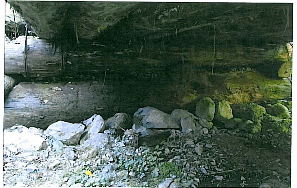
CK-2406 Left abutment
