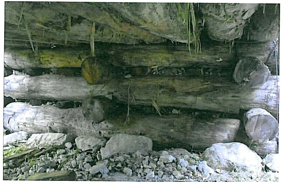
CK-2406 Right abutment
